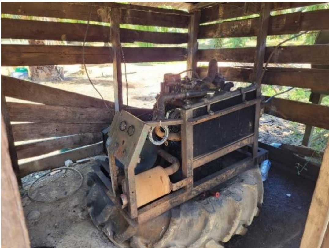
Figure 1.1: Diesel Generator in Peladang Sandakan
