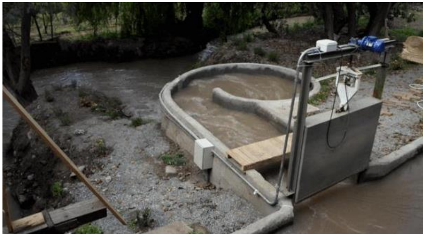
Figure 2: A General Gravitational Water Vortex Power Plant
