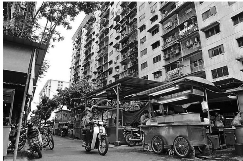
Figure 2: The Rifle Range Road Flats in Penang
