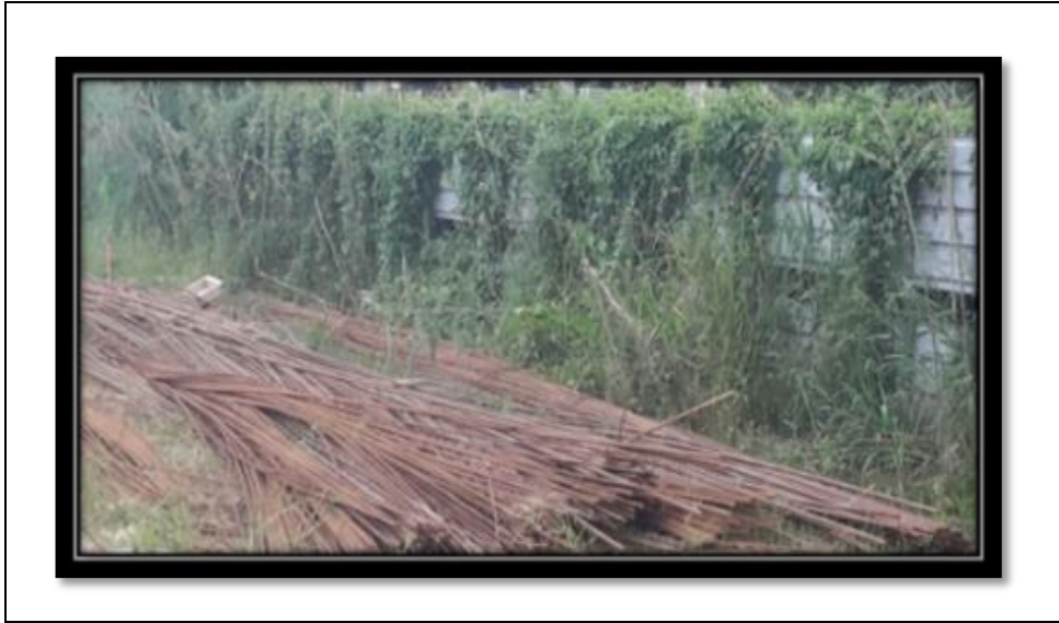
Figure 1.1: Corroded High Yield Steel Bars laid on the Ground
