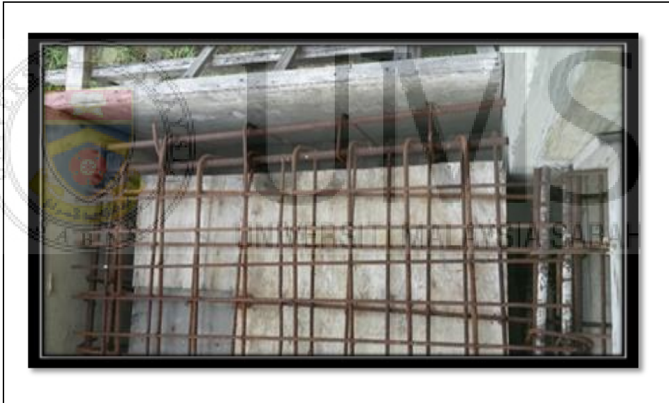
Figure 1.2: Corroded Reinforcement
