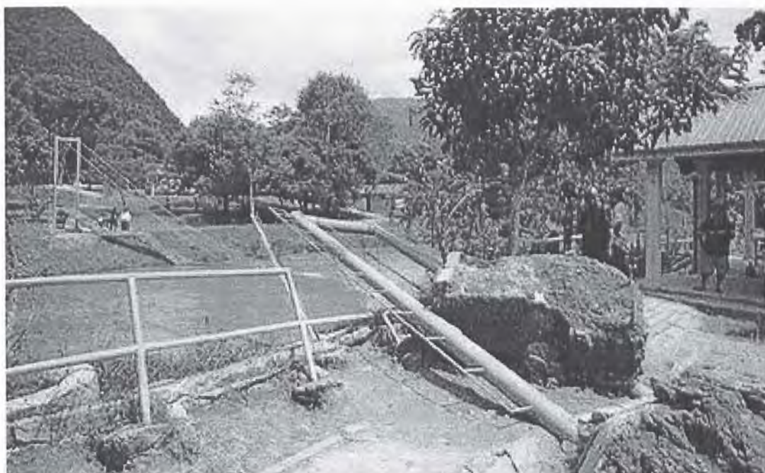
Figure 1.3: Suspension Bridge Collapse at Kuala Dipang, Perak (26/10/2009)
